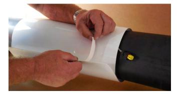
Remove adhesive strip and seal cover tightly.
