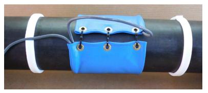
Hold Pipe Cover up to Install area and mark length. Install weather stripping inside the line at each end.
